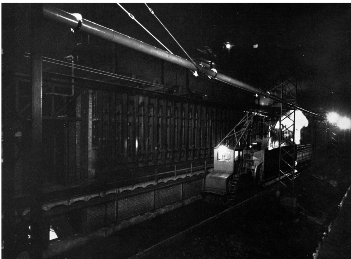
A night-time view of one of the two Woodall Becker Compound carbonisation oven batteries. Each had 53 ovens, in side-by-side banks. The works were expected annually to carbonise about 750,000 of coal, producing 500,000 tons of solid smokeless fuel for domestic use and over 5,000 million cubic feet of town gas (i.e. gas from the carbonisation process).
